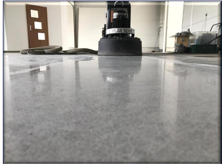
We recommend the **HTC SuperFloor™ Bronze** polished concrete surface for all flooring where the surface is perfectly smooth or where a **HTC SuperFloor™** concrete sanding technique has already been used. All this with only a few polishing steps, in a quick and efficient way. It is much more resistant to external impacts than surfaces with other coverings. It allows a smooth rolling not only for forklifts and pallet trucks, but also for all wheel-mounted equipment.
